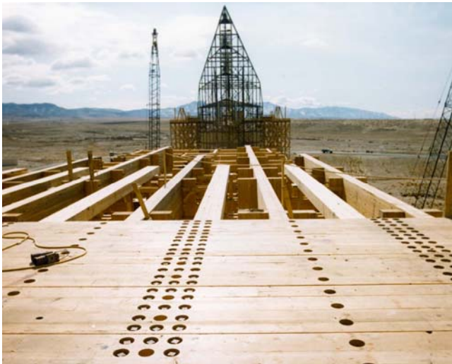
Figure 18: Detail of the deck construction
