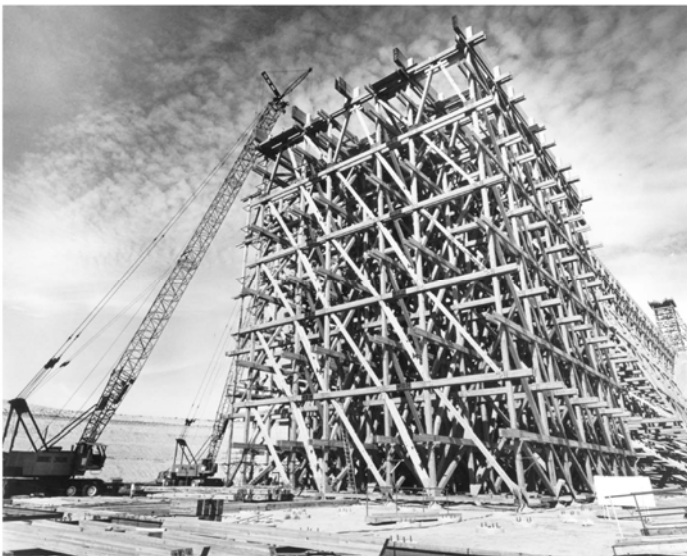
Figure 17: TRESTLE during construction
